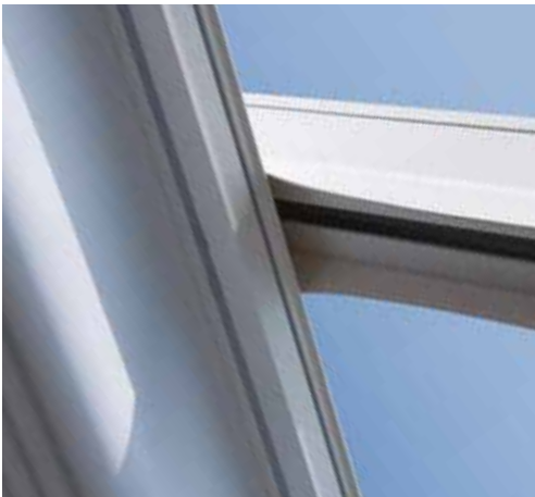
when the width exceeds 4,5m : with extra guide in the middle
